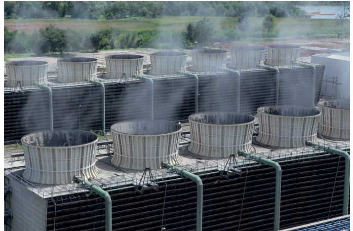
Typical open cooling towers
